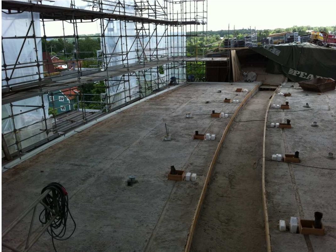
Figure 11 Removed roof structure exposes cavities and holes for rain and moisture, Emilsborg 3.
