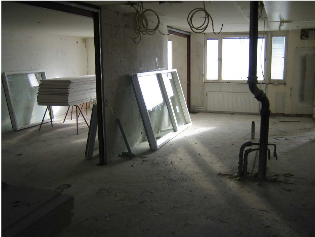
Figure 14 Openings of bearing wall to obtain a more spacious layout, Fredslyckan.
