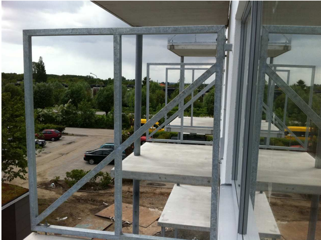
Figure 15 Inclined steel strut anchors the balcony to the building, Fredslyckan.
